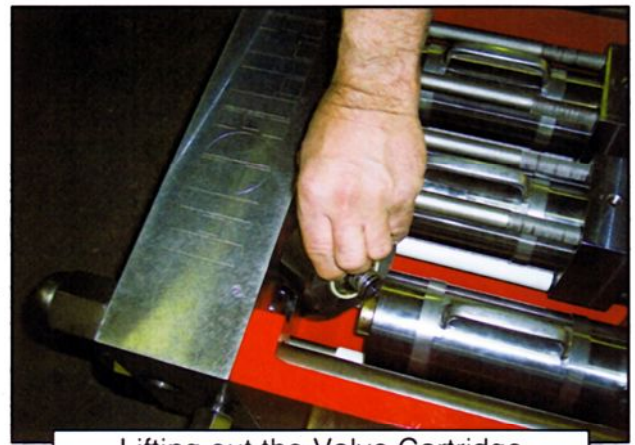
Lifting out the Valve Cartridge
